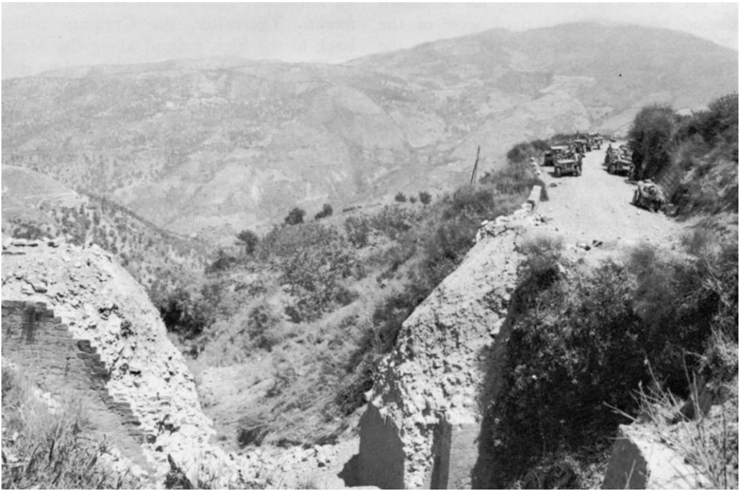
DEMOLISHED BRIDGE ALONG HIGHWAY 117 between Santo Stefano and Mistretta slows down 45th Division troops.
