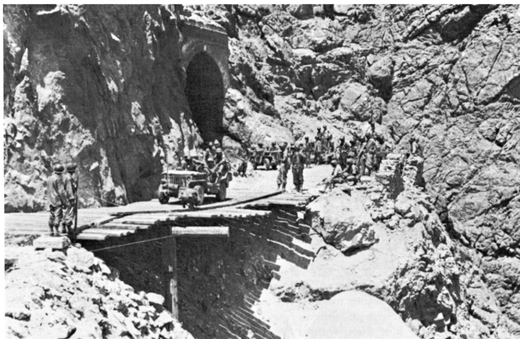
THE BRIDGE THAT WAS "HUNG IN THE SKY" BY THE 10TH ENGINEER BATTALION
