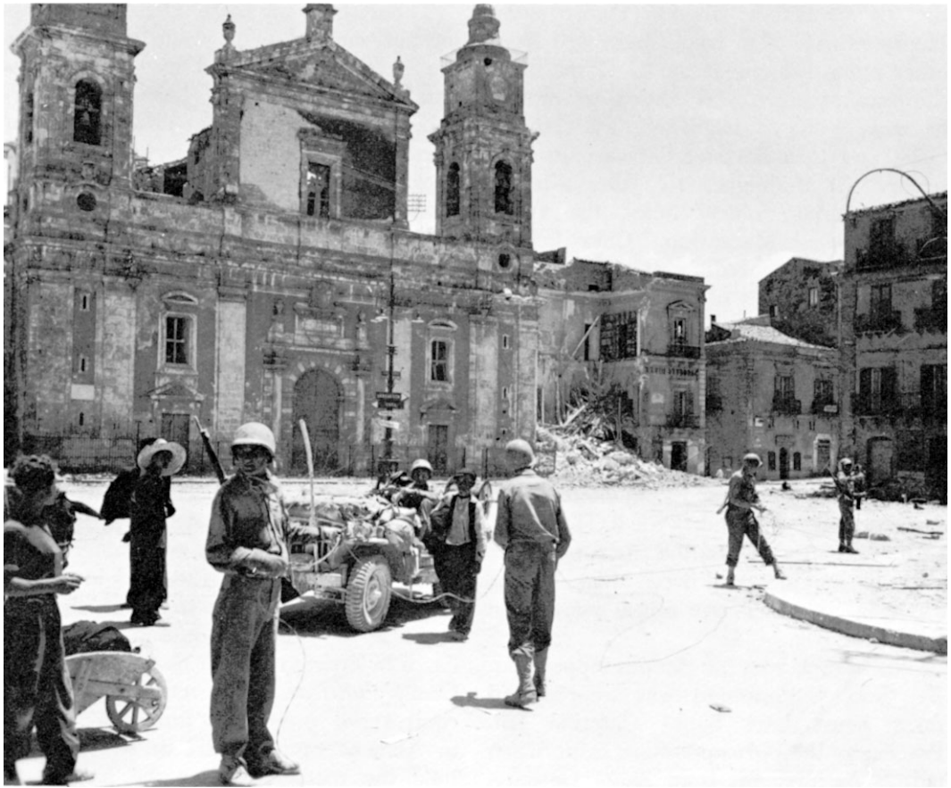
SIGNAL CORPS LINEMEN setting up wire installations in Caltanissetta, 18 July.
