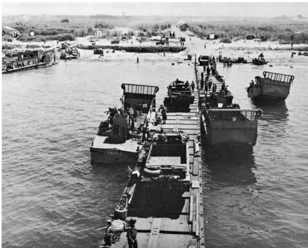
LANDING HEAVY EQUIPMENT over the causeway at Scoglitti.
